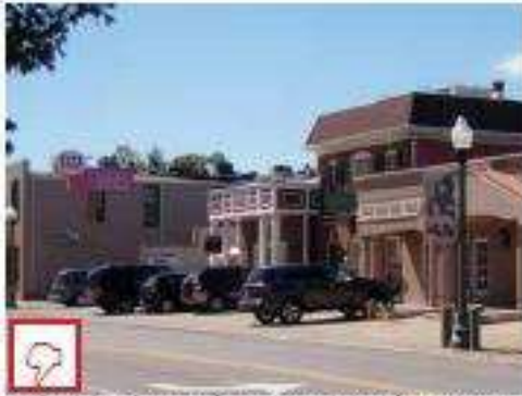
Head-in parking along street frontage is inappropriate for Downtown. Drive; note how the vehicles block the sidewalk and force pedestrians to unsafely walk in the street.
