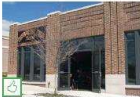
Low-pitched roofs are permitted and shall present a parapet wall at the building facade; note the simple, and appropriate, brick soldier cornice.
