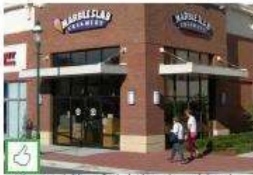
Metal canopies shall have a finished ceiling and may only be set between the storefront head and transom window sill
