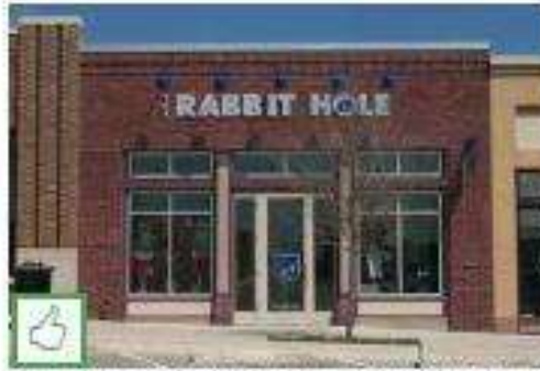
This simple one-story façade wall includes a detailed brick cornice cap and horizontal façade bay articulation with columns in the storefront.
