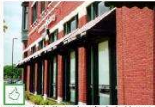
Awnings may be placed between the storefront head and the transom sill
