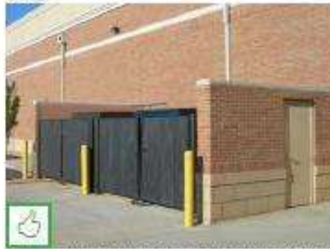
This dumpster area is appropriately located to the rear of the building and enclosed with a screen wall; note the screen wall materials are coordinated with the building.
