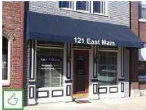
This simple shed awning is an appropriate awning style for Downtown Erwin; note the appropriate scale, coordinating color and the correct placement of the awning above the storefront entry.
