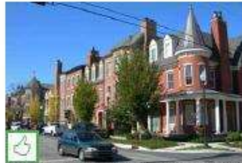
This street wall illustrates a variety of ways to appropriately detail roof forms for townhome transitional buildings; note the appropriate use of dormers and a corner porch and tower element at the street corner.
