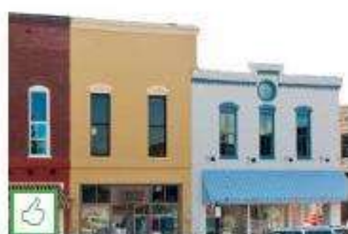
Vertically proportioned windows that exceed the 2:1 ratio are appropriate for upper stories
