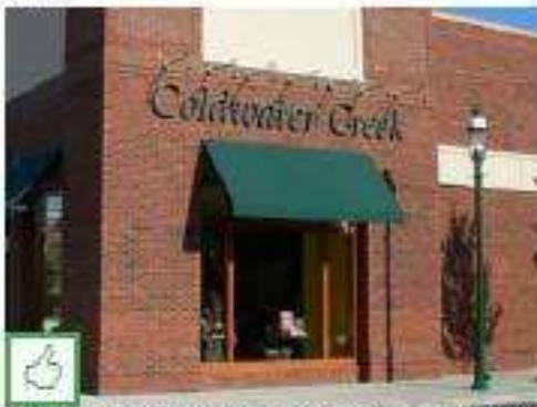
Indirectly illuminated individual letters and graphics are appropriate types of wall signs; note appropriate placement above storefront.
