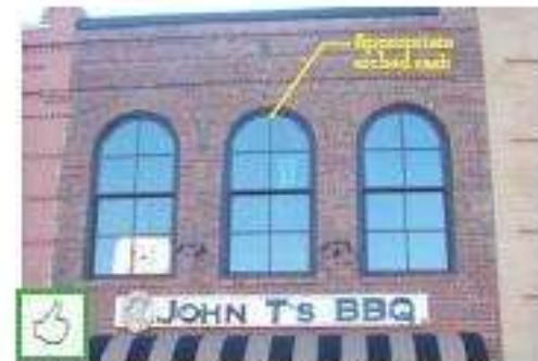
Arch-top sashes are appropriate; note appropriate four-over-four muntin pattern
