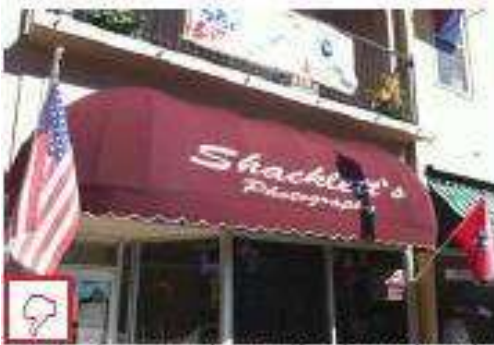
Dome shaped awnings are only permitted for arch-top windows and doors and shall be sized to match the opening
