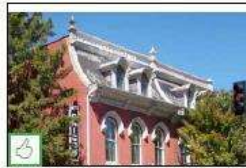
Appropriately detailed mansard roofs that are integrally designed as part of the building are permitted; note the slate shingles and dormers.
