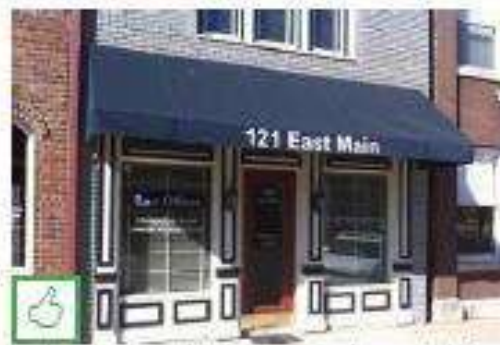
Simple shed awnings are historically accurate and are permitted either with or without a valance or end panels
