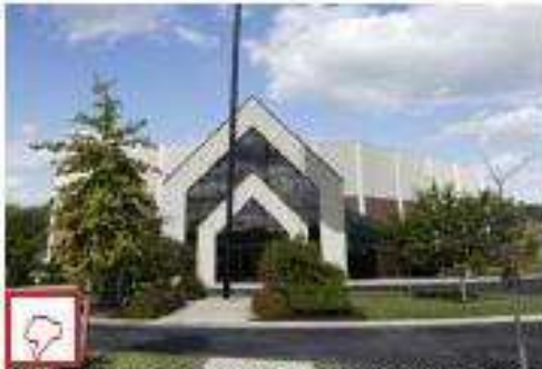
This sanctuary building lacks appropriate massing detail; it presents a facade of large, flat, windowless walls and is surrounded by a large parking lot on all sides.
