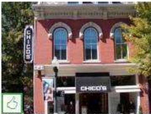
Indirectly illuminated blade signs are appropriate for upper floor placement only on building corners; note the appropriate scale and craftsmanship of the sign.
