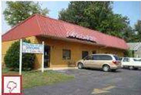
This metal, overhanging bite-mass roof is inappropriate for downtown Erwin; note also the inappropriate use of painted concrete block as a facade material.
