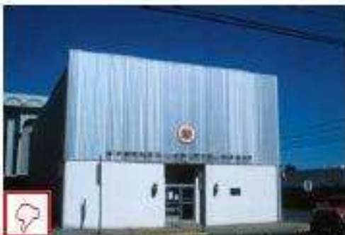
This civic building lacks appropriate facade detailing and windows and is clad inappropriately with industrial metal siding and L.F.S.
