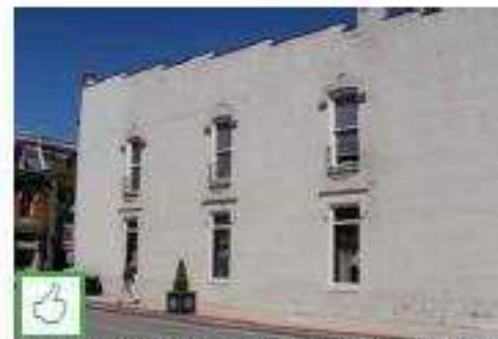
Parapets are permitted to step along facade walls of corner buildings fronting secondary streets to match roof pitches.
