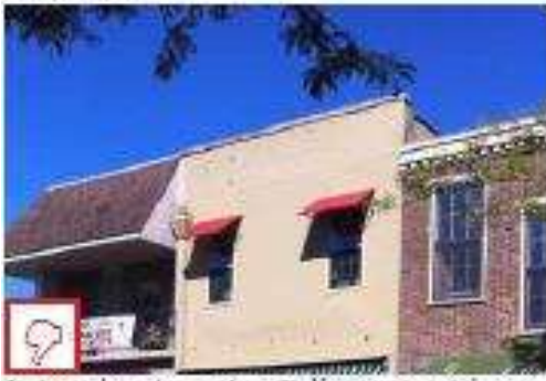
Awnings and canopies are not permitted for upper story windows
