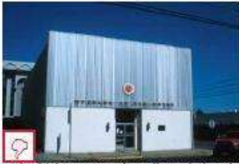
Façade walls lacking appropriate architectural horizontal and vertical articulation are not permitted.
