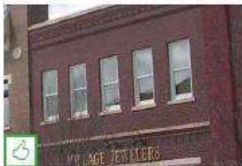
Vertically proportioned windows (2:1 minimum) are appropriate for the upper stories of new buildings in Downtown Erwin
