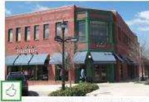
This two-story corner façade includes an appropriately detailed corner entry bay and brick cornice detailing.
