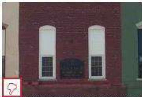
Vinyl residential windows and any windows inappropriately sized for the original masonry opening are not permitted
