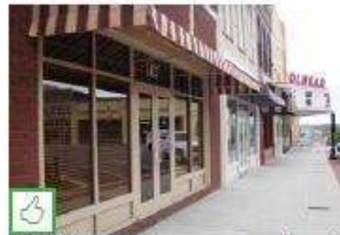
Pre-finished aluminum storefront systems are appropriate for ground floor office uses as the building may change to a retail use in the future.
