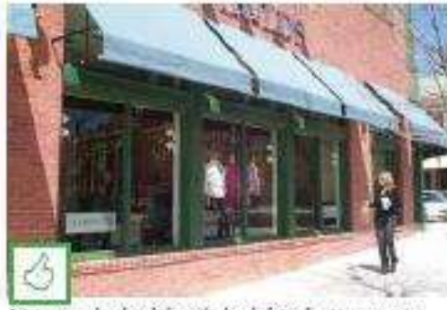
Awnings may be placed above the head of storefront transom windows; note appropriate size for window bays
