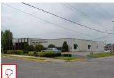
This municipal utility office building lacks appropriate facade detail and inappropriately places the parking lot and drive-thru lane at the street corner; note the lack of a sidewalk on the secondary street.
