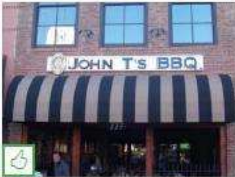
This well-crafted, exterior illuminated panel sign is appropriately located between the storefront transom window heads and the sill of the second story window.
