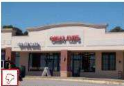
Parapet walls shall align with the building facade wall; this strip mall roof inappropriately protrudes beyond the facade wall.
