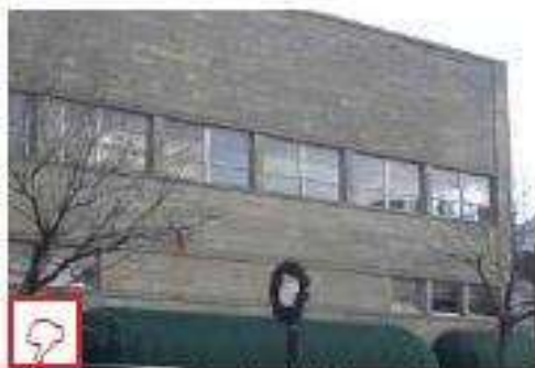
Horizontally proportioned windows and "ribbon windows" are inappropriate for upper stories in Downtown Erwin
