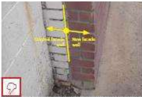
Original building façade walls shall not be covered or encapsulated with new brick veneer facades.
