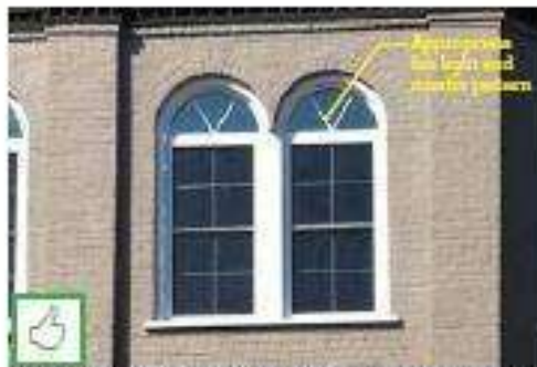
Muntin patterns of four-over-four or less are appropriate for windows of commercial/mixed-use buildings in Downtown Erwin; note the appropriate 3-light fan pattern
